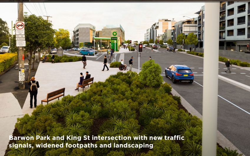
St Peters Square looking south - with new separated cycleways, widened footpaths, dynamic community spaces and landscaping
