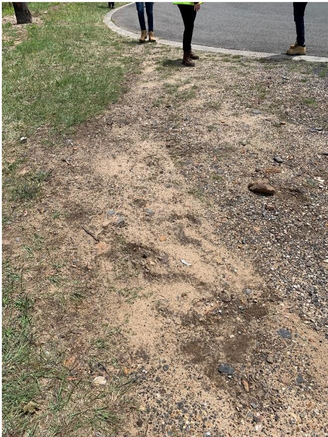
*Photo 7: Evidence of fill making its way through the drainage system and conduit that potentially contains asbestos. Location is between Great Western Highway and Medlow Bath Station (looking West).*
