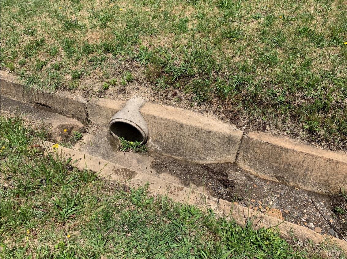
*Photo 8: Example of existing stormwater pipe potentially containing asbestos (looking West)*
