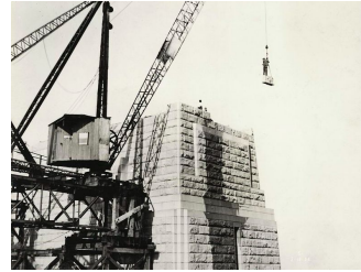
Lifted Masonry for Pylon Tower
