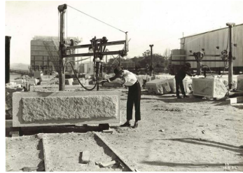
Dressing Granite Blocks
