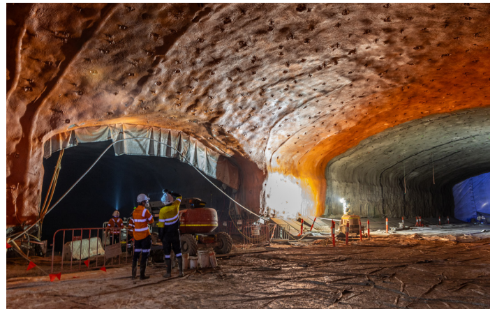
First layer of water proofing at Arncliffe, January 2024
