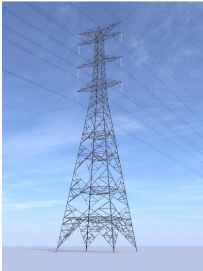
Plate 11: Example of transmission line towers
