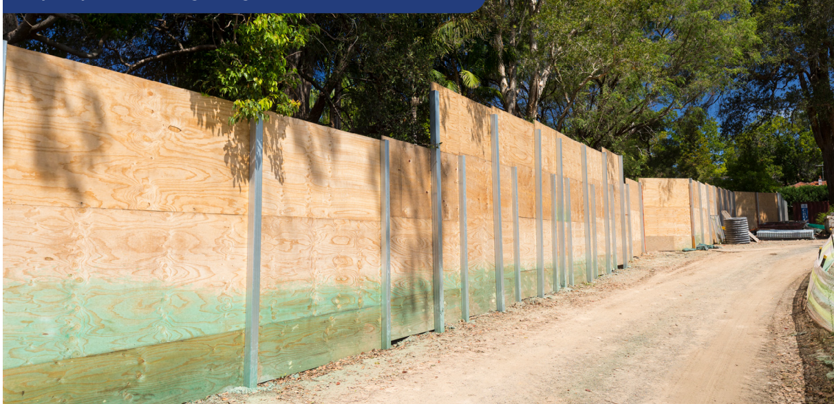
Temporary noise hoarding during construction of NorthConnex
