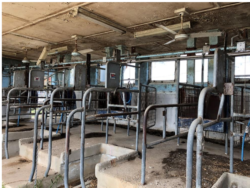
Figure 33: The abandoned dairy, McGarvie Smith Farm 2020 (Source: S Graham TfNSW)
