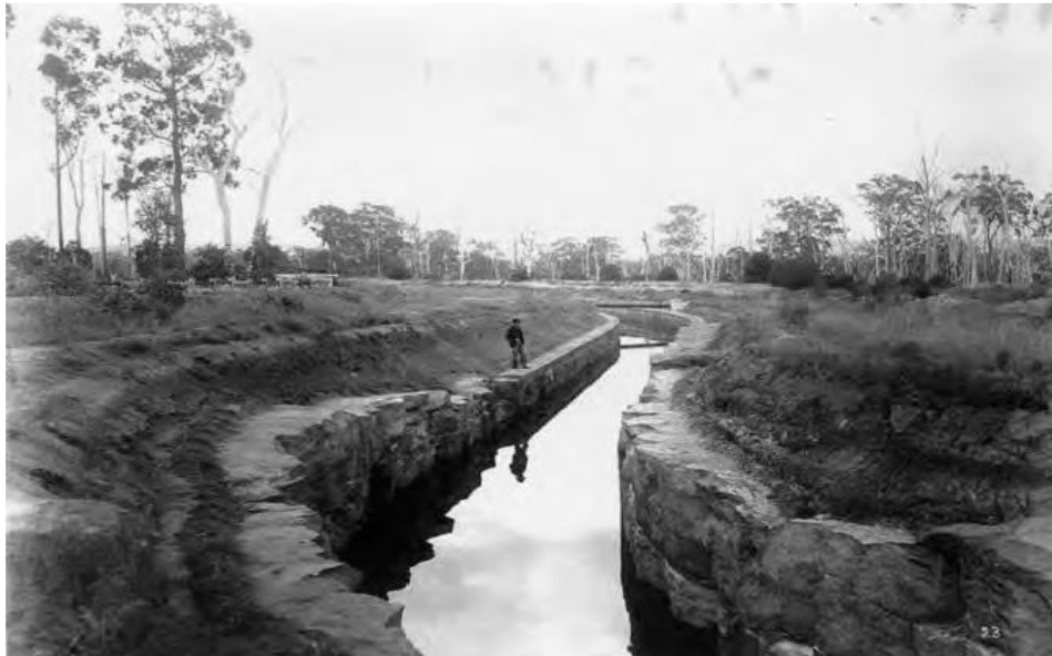
Figure 14: a rock cut and masonry lined section of the Canal c1898 with flume in the background and showing the serpentine nature of the Canal system 66
