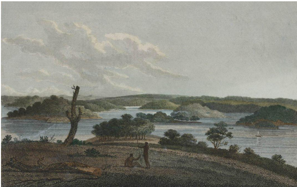
Figure 3: Sketch by J. Heath, By water to Parramatta, with a distant view of the western mountains , taken from the Windmill-hill at Sydney, 1798 (Source: Dixson Library, State Library of NSW)
