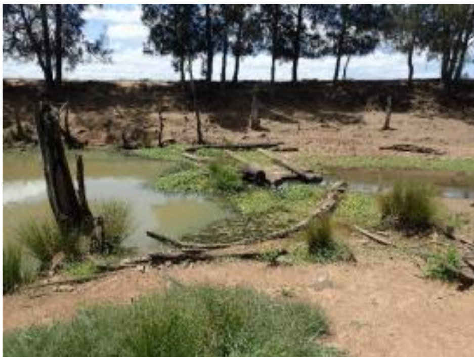
Figure 13: Remains of the original South Creek Bridge, 2019 (Source EIS Section 7.6, p. 536)
