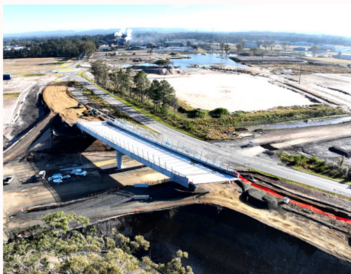
Progress on bridge barriers, safety screens and batter treatments at Masonite Road overpass bridge
