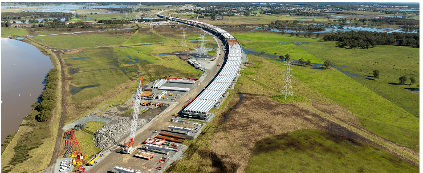
Construction of 2.6-kilometre viaduct progressing from Tarro to the Hunter River
