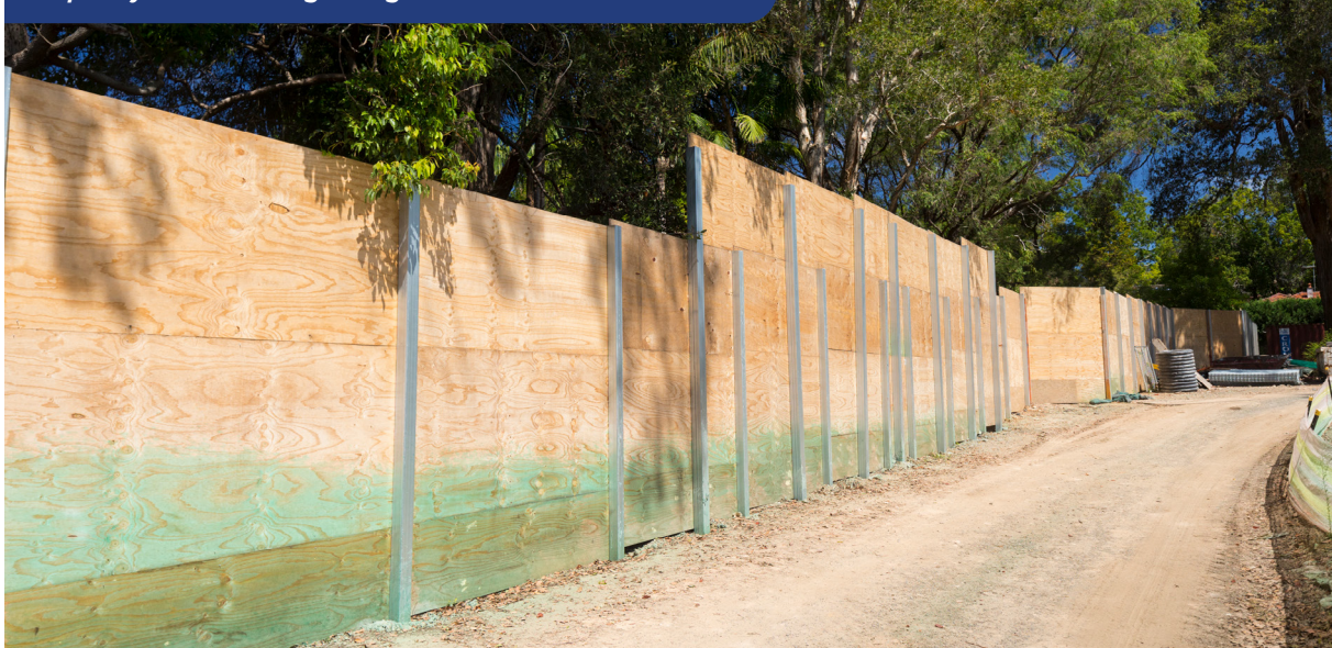
Temporary noise hoarding during construction of NorthConnex
