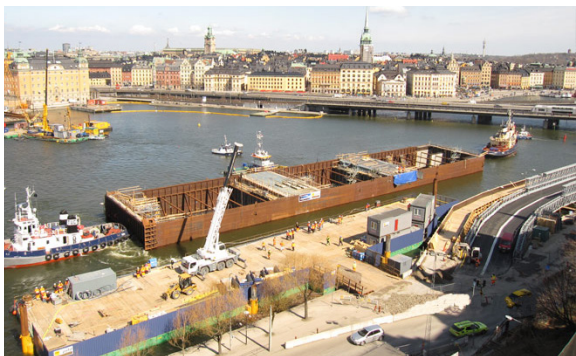
3. Floating steel shell unit arriving at casting facility for concrete construction.
