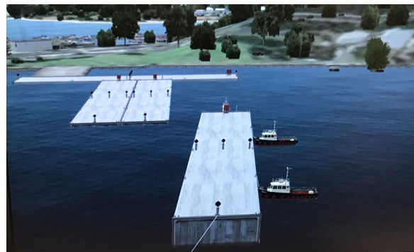
2. Steel shell unit arrives at construction site casting facility.
