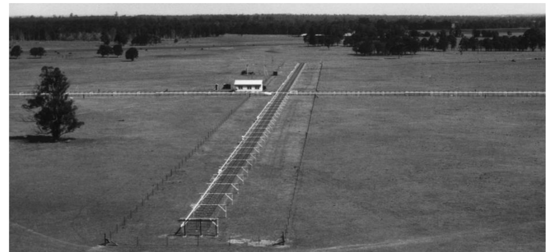
Figure 20. View looking south showing the N-S arm and most of the E-W arm of the Mills Cross, with the receiver hut at the centre of the array. Source: ATNF Historic Photographic Archive (3476-3).
