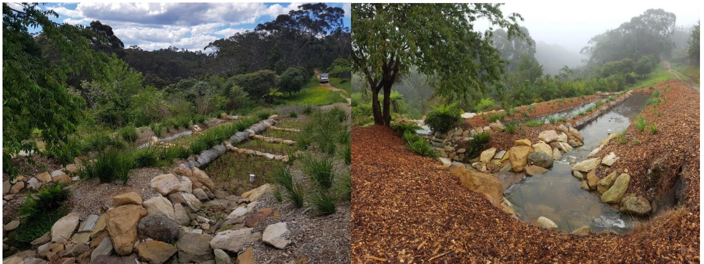
Figure 3-12: Indicative treatment at basin outlet (source: Blue Mountains City Council)
