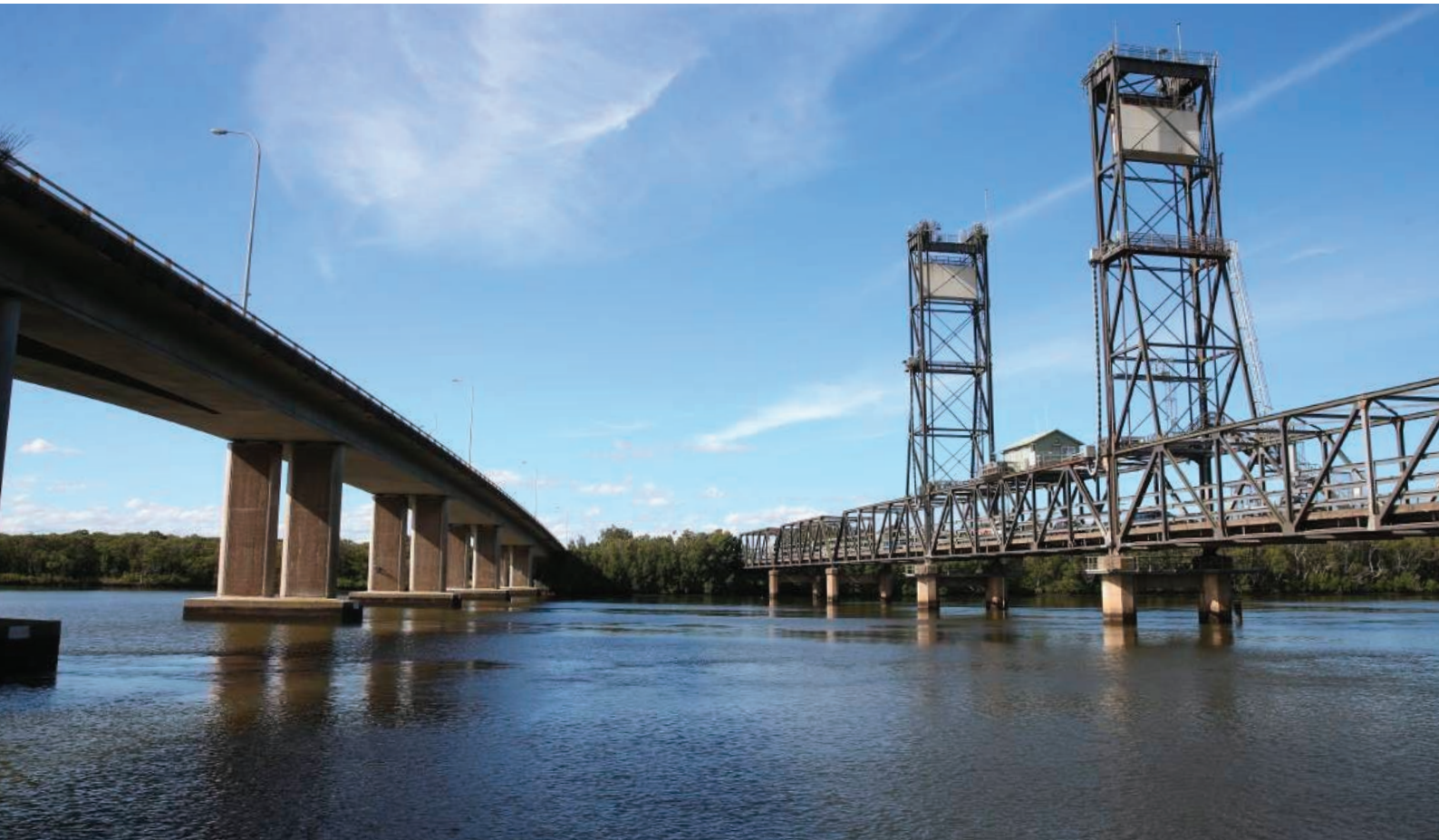
Hexham Bridge over the Hunter River
