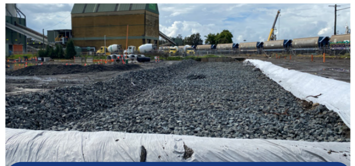
Localised controls within site to capture sediment
