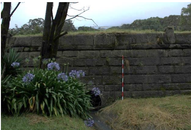
Figure A-19: local heritage item ‘Road culvert and sustaining wall at Emoh’ looking northward
