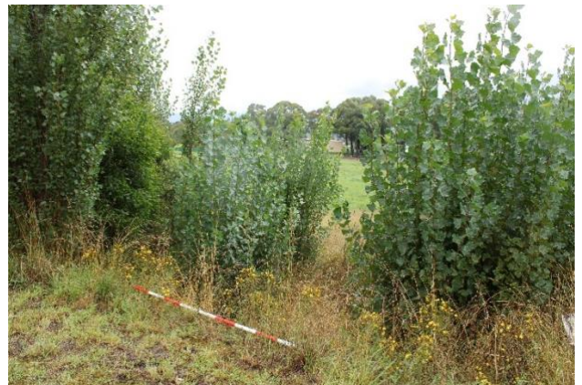
Figure A-24: Modern concrete culvert, vegetation restricted access and visibility. Looking downhill from southern side Highway verge
