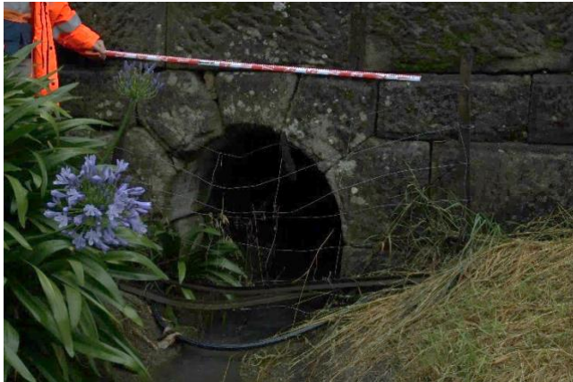
Figure A-21: Culvert at the base of the stone wall
