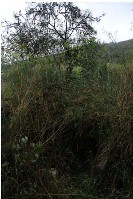
Figure A-30: Modern concrete culvert (obscured by vegetation) located on western side of the Highway
