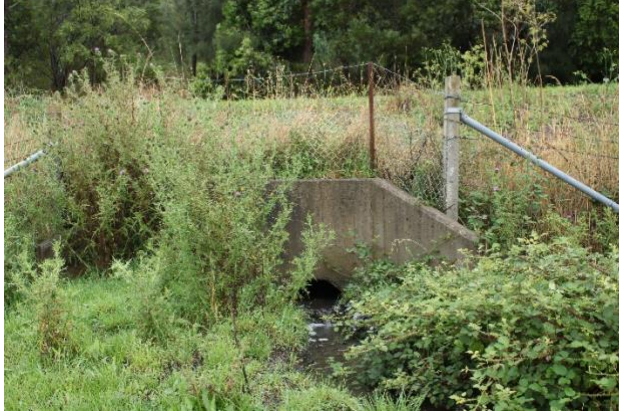
Figure A-25: Modern concrete culvert located within the curtilage of local heritage item 'Umera', looking north from the paddock adjacent to the item
