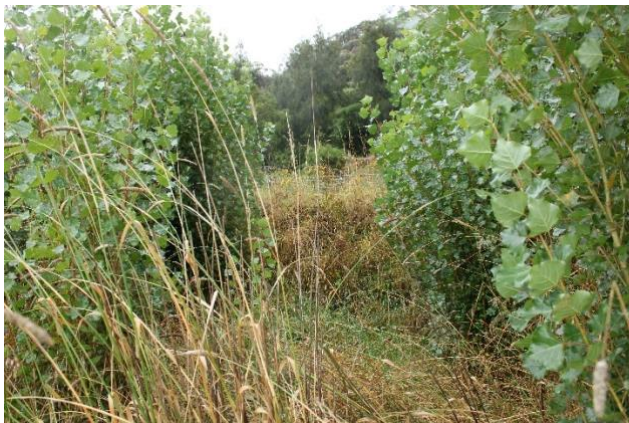
Figure A-23: Modern concrete culvert, vegetation restricted access and visibility. Looking north with Highway above
