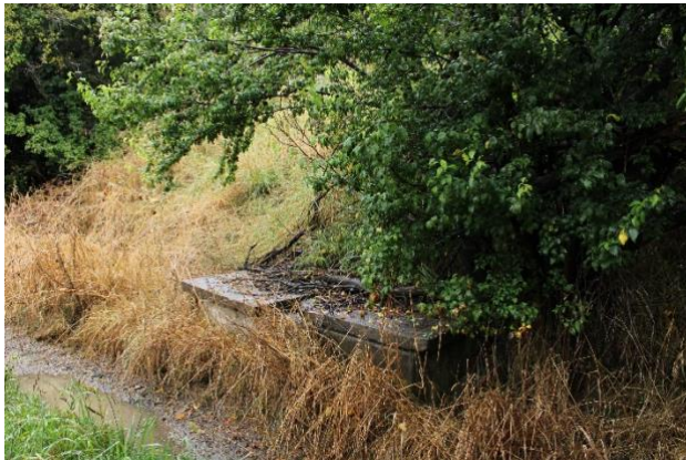
Figure A-27: eastern side of the culvert alongside the old highway alignment. Covered over with modern concrete casing – partially visible due to vegetation.
