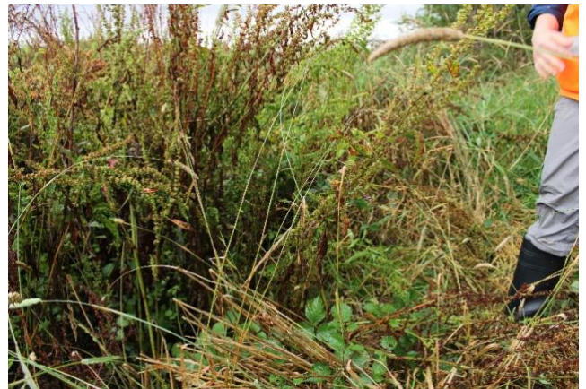
Figure A-31: Modern concrete culvert (obscured by vegetation) located on western side of the Highway
