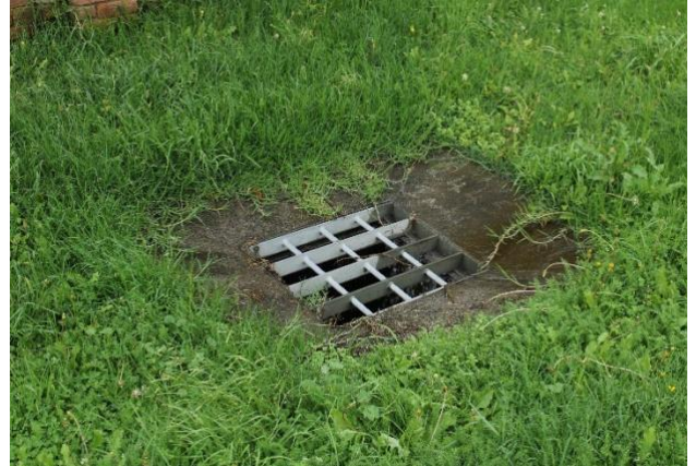
Figure A-33: Close view of one of the two modern concrete and metal culvert along the road verge on the eastern side of the Highway
