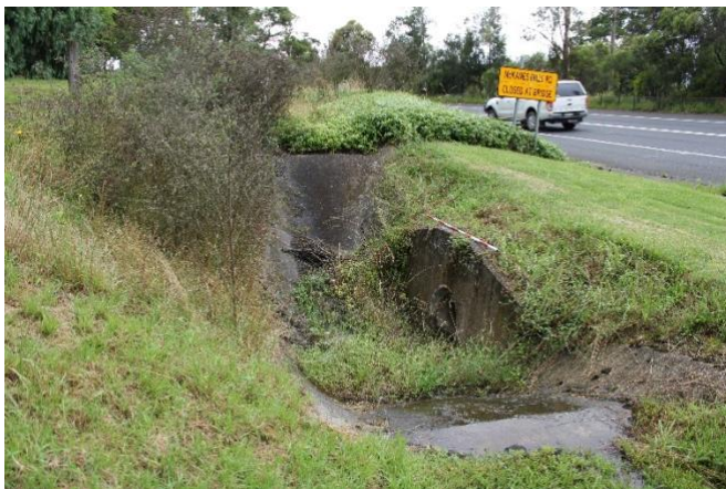
Figure A-34: Modern concrete road culvert on the eastern side of the Highway at 3462 Great Western Highway
