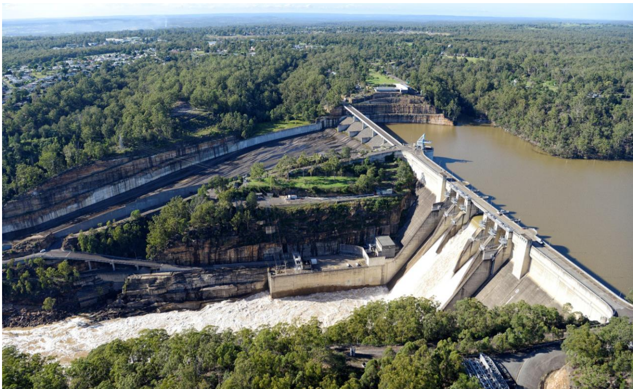
Figure 8. The existing Warragamba Dam during a flood
