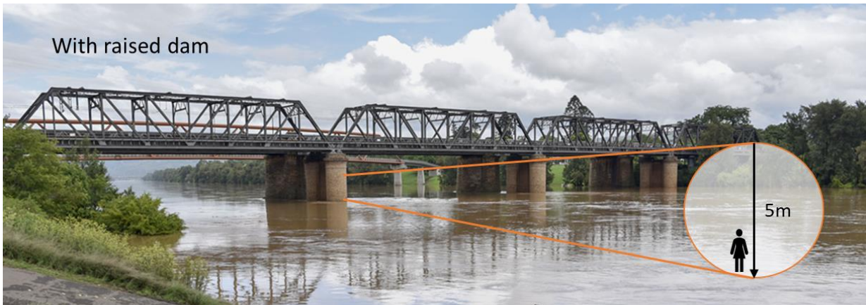
Figure 21. The Victoria Bridge at Penrith with levels five metres lower than March 2021 flood peak – equivalent to the reduction with the raised dam
