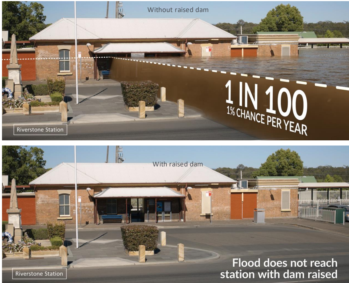
Figure 23. Riverstone Station in a 1 in 100 chance in a year flood – without and with the raised dam
