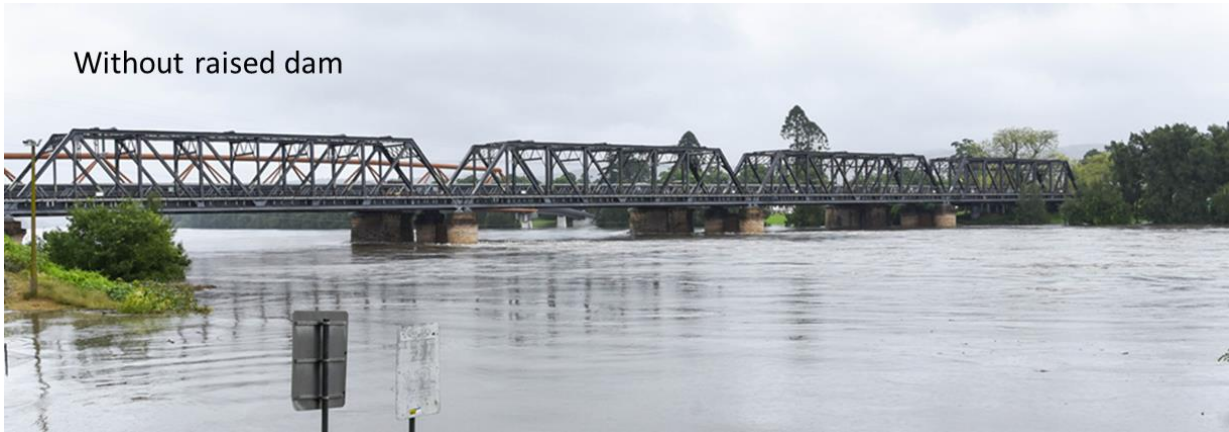
Figure 20. The Victoria Bridge at Penrith near the peak of the March 2021 flood
