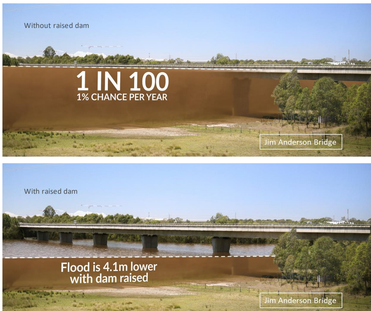
Figure 22. The Jim Anderson Bridge at Windsor in a 1 in 100 chance in a year flood – without the raised dam (top) and with the raised dam (below)
