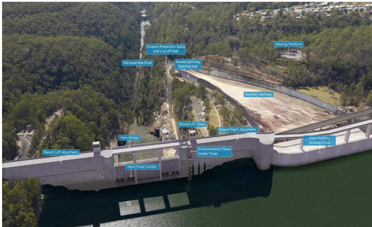
Figure 12. Artist's impression of the upstream face of the raised dam
