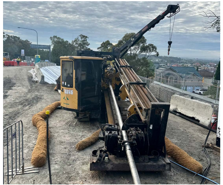
HDD machine on Elizabeth Drive to relocate underground gas.
