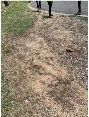
Photo 7: Evidence of fill making its way through the drainage system and conduit that potentially contains asbestos. Location is between Great Western Highway and Medlow Bath Station (looking West).
