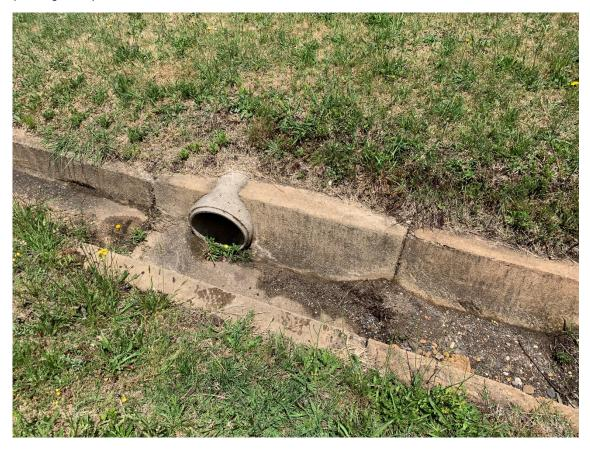
Photo 8: Example of existing stormwater pipe potentially containing asbestos (looking West)
