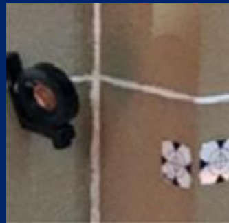
Survey targets on the façade of a building
