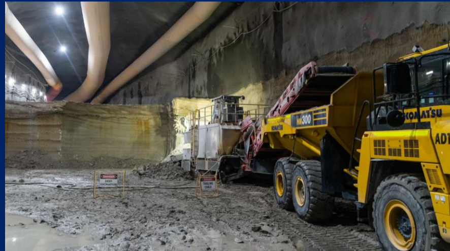
Deep bench excavation
