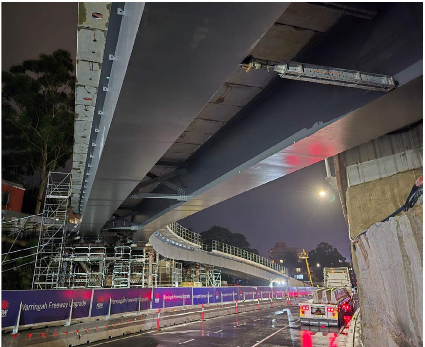
Picture 1: The new Falcon Street southbound bus on ramp after the installation of girders over the southbound outer lanes of the freeway.
