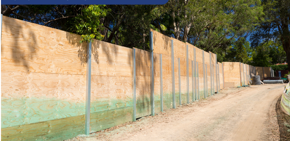
Temporary noise hoarding during construction of NorthConnex
