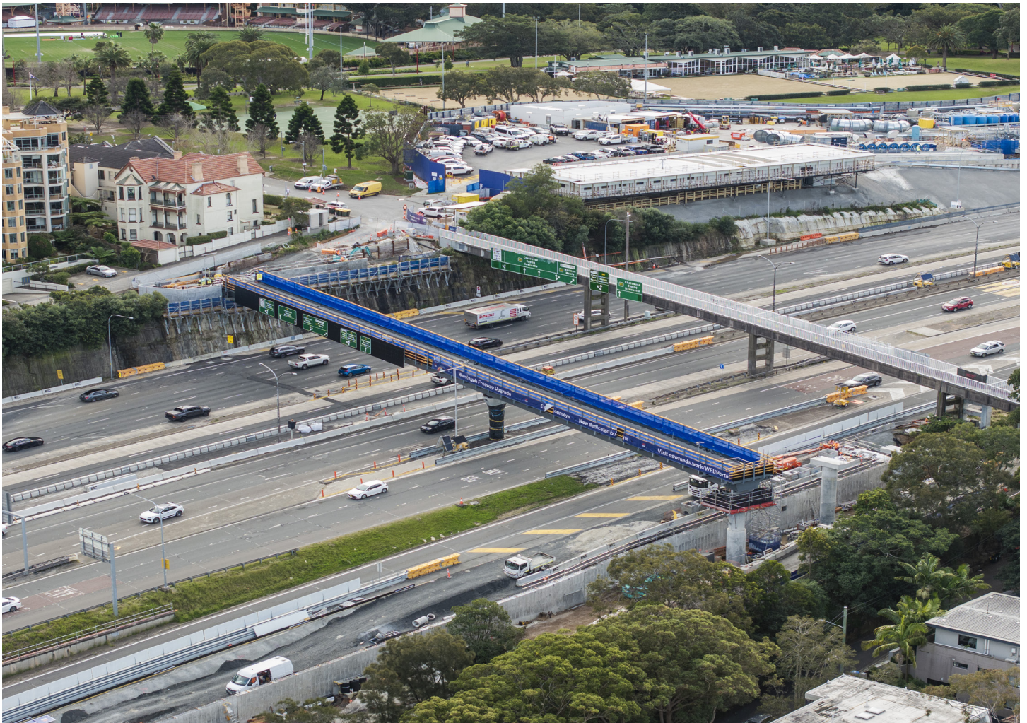
Image: New Ridge Street shared user bridge and existing Ridge Street shared user bridge photographed in July 2024.
