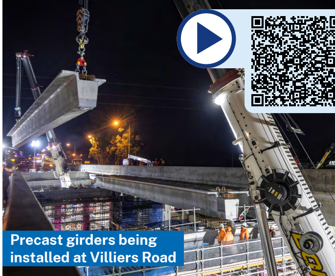
Precast girder installation
