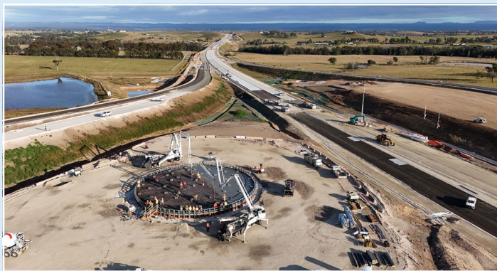
All in a days work: pouring the concrete base
