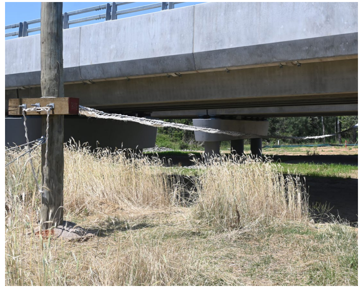
Fauna rope crossing under the new Kemps Creek bridge
