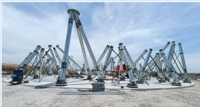
Installing the steel columns
