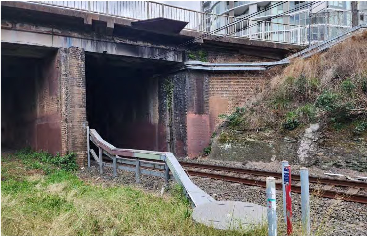
Figure 1-6 View of Epping Bridge looking north from the rail corridor
