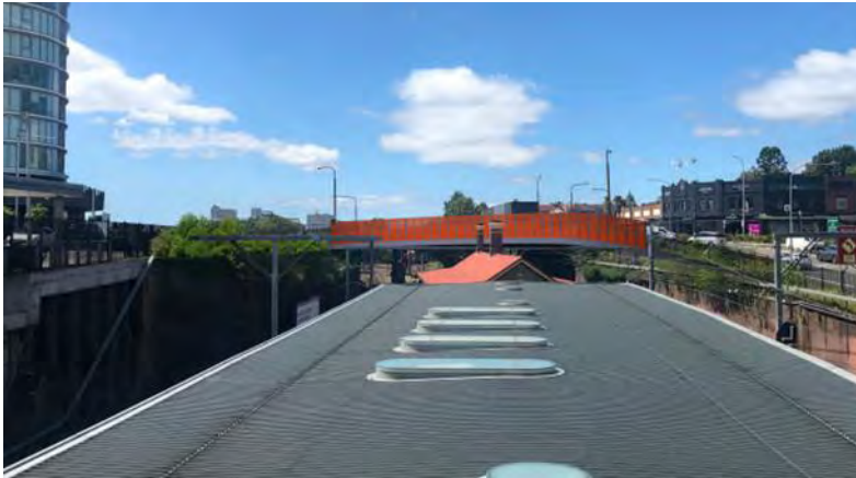
Figure 6-14 VP1 from Epping Station existing and proposed (indicative only, subject to detailed design)
