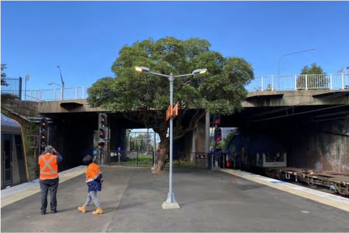
Figure 1-5 View of Epping Bridge looking south from Epping Station
