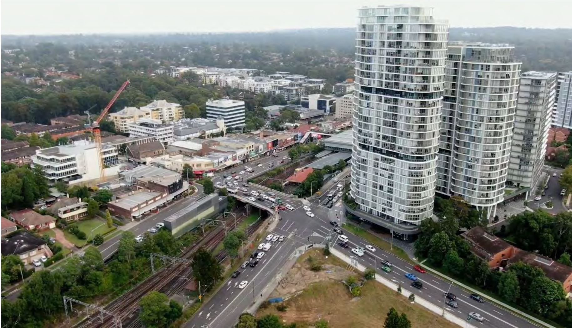
Figure 1-3 Aerial image of Epping Bridge (Transport, 2024)
