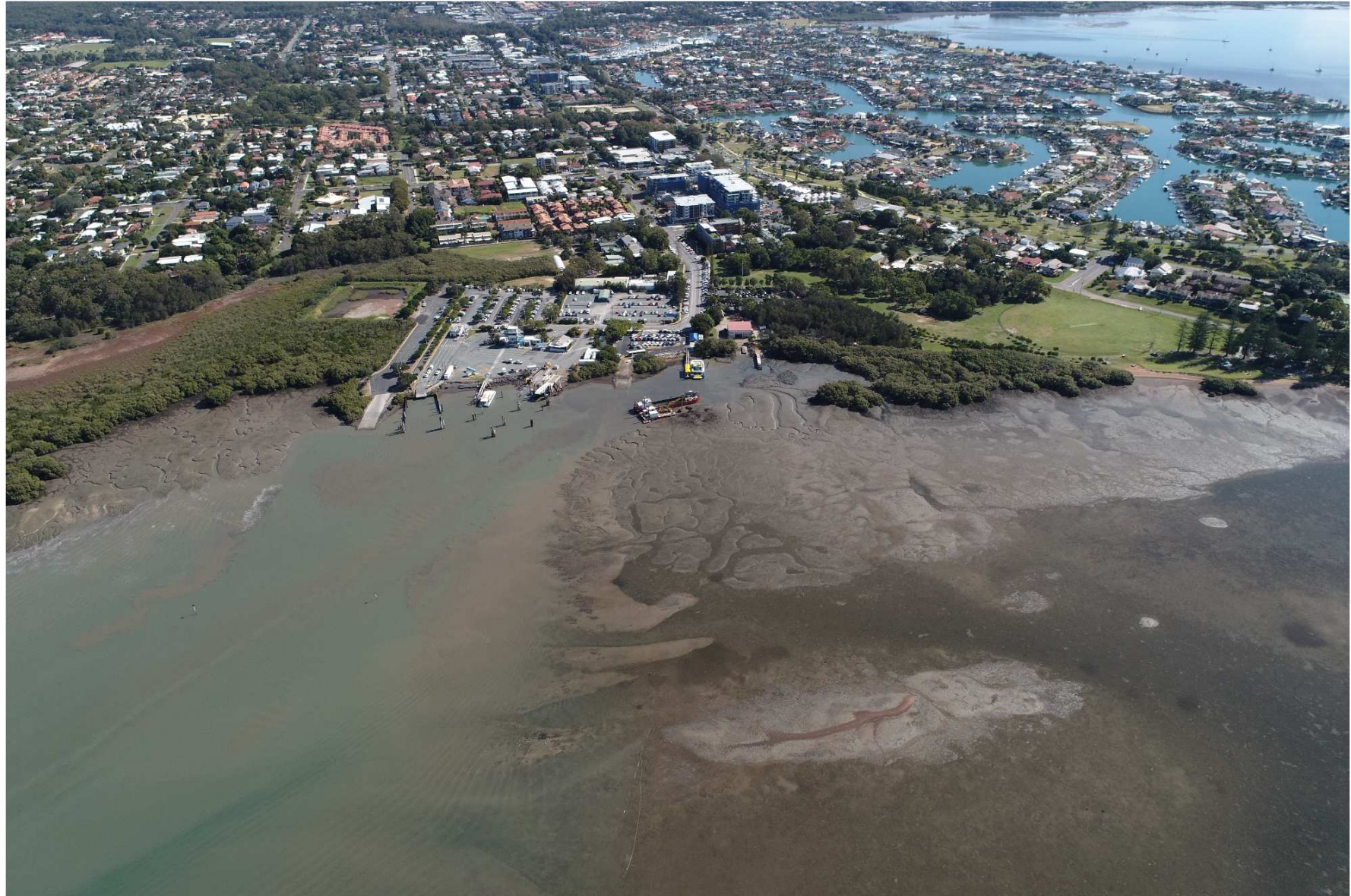
Plate ES-1: Toondah Harbour
