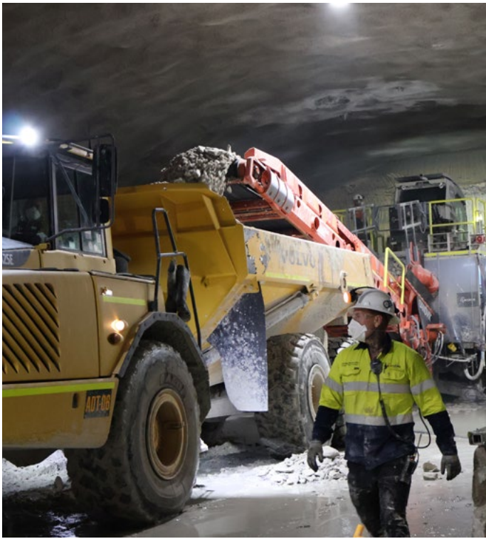
Roadheader tunnelling activities at Cammeray
