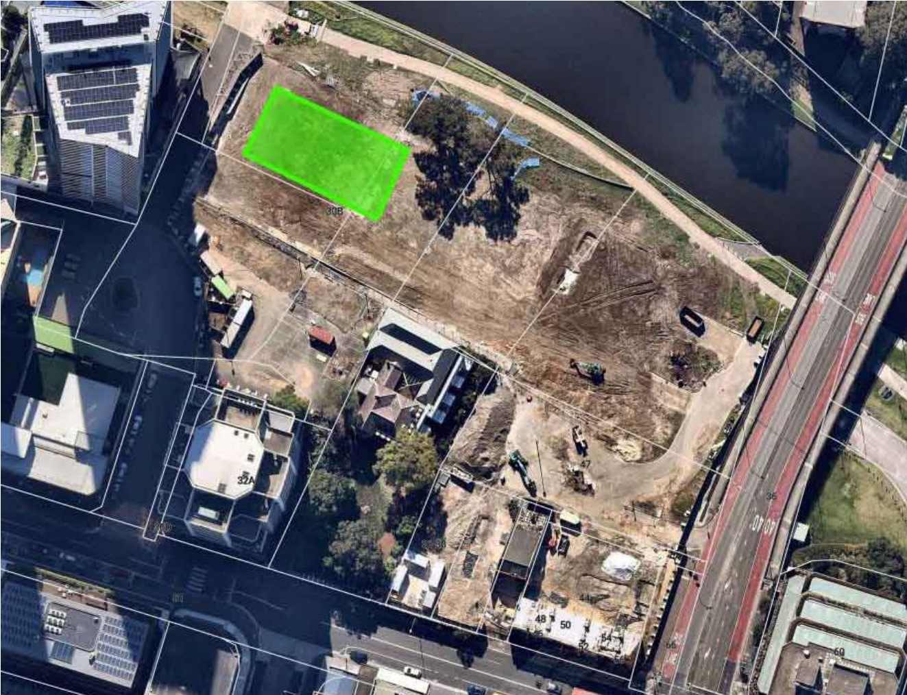
Figure 4-1 Area in green indicates the area remaining to be monitored during excavations.
