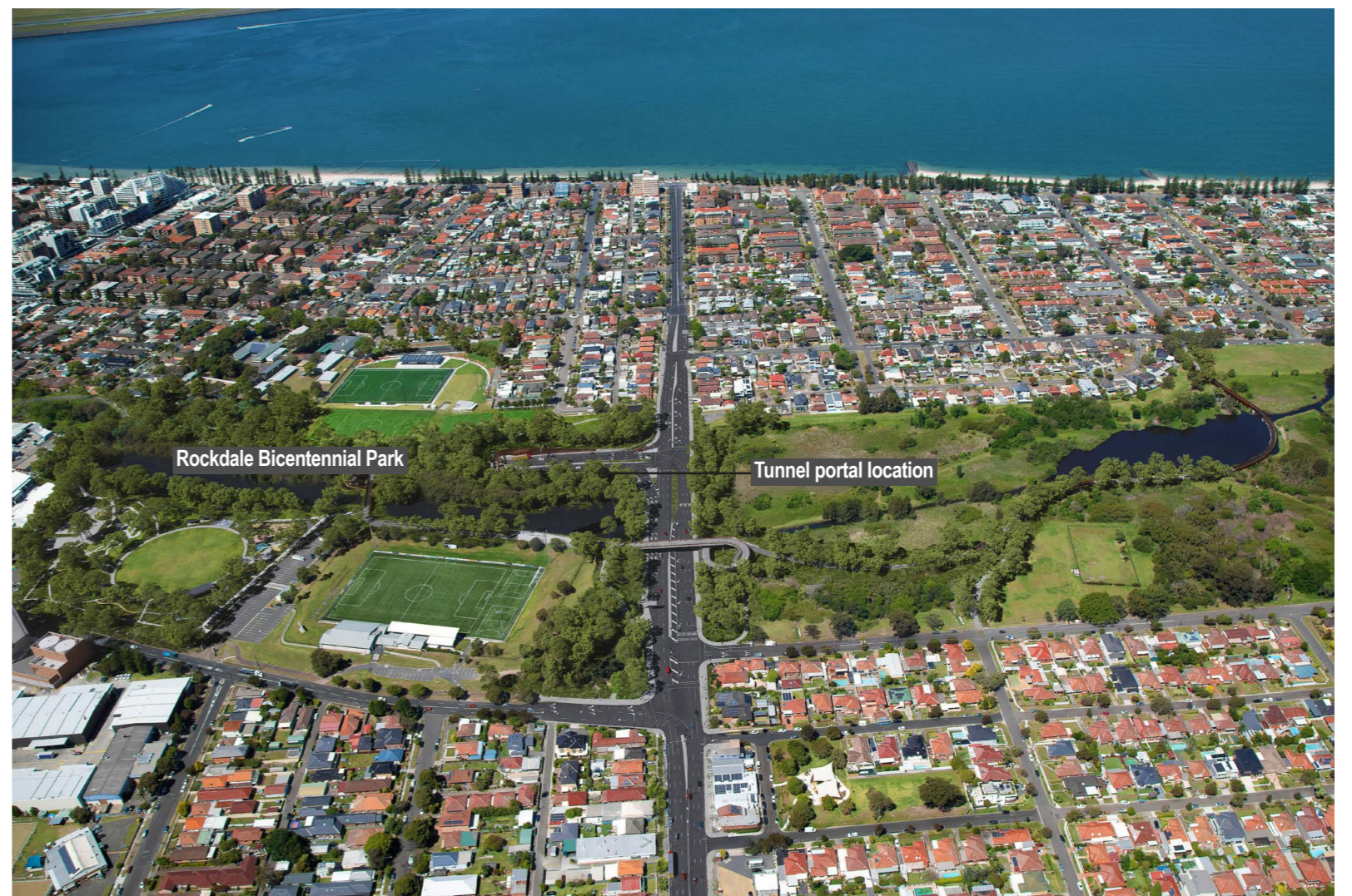
Aerial photo over President Avenue looking east to Botany Bay with approximate tunnel portal location shown
