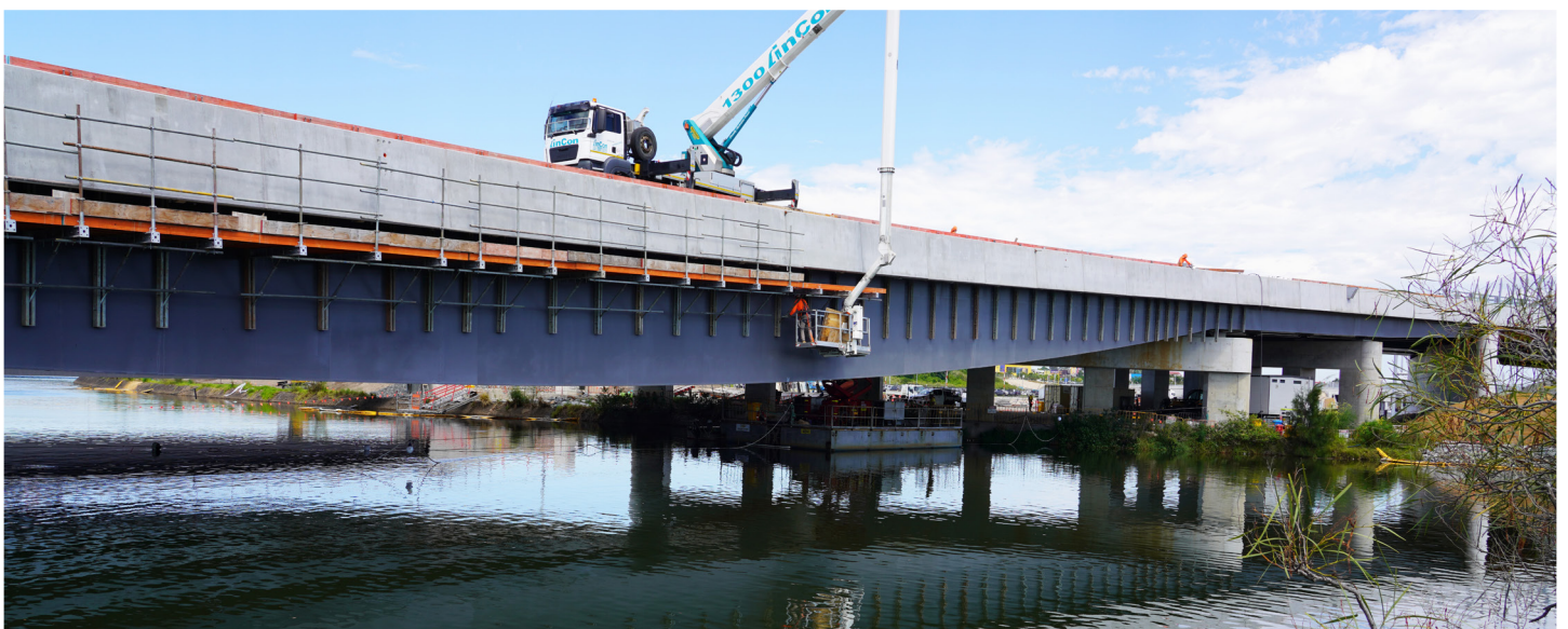
Installation of utilities services under some of the bridges across the Alexandra Canal.
