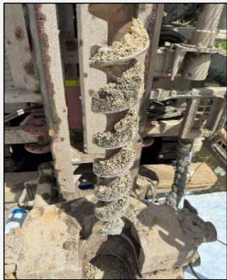
Photo 8: 16/01/2024: Representative image of soil material (BH154)
