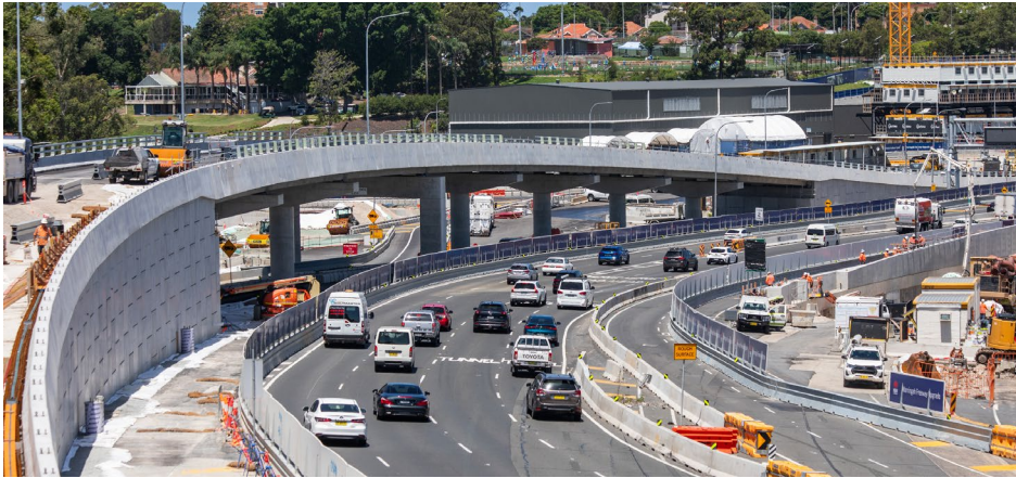
Progress on the on Miller Street ramp, January 2025.
