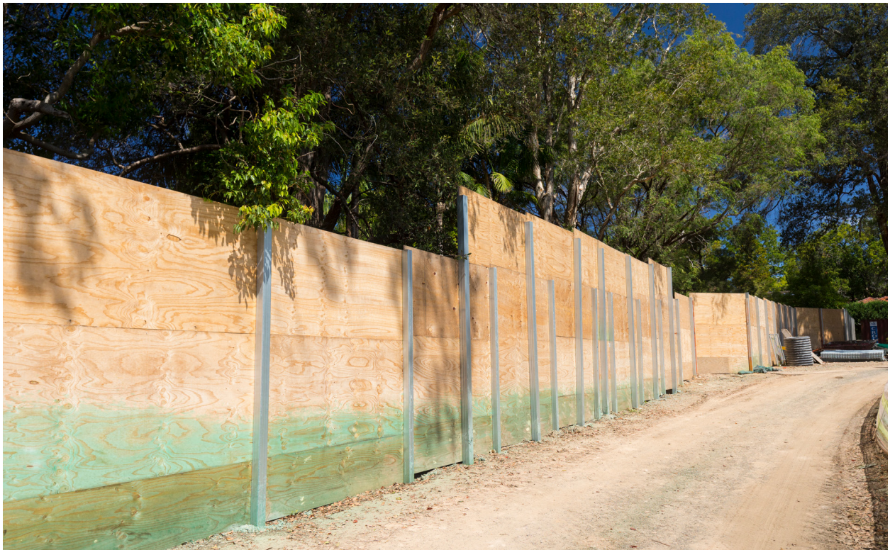
Temporary noise hoarding during construction of NorthConnex
