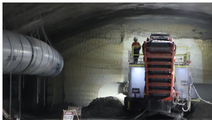
Roadheader excavation from the Cammeray site.
