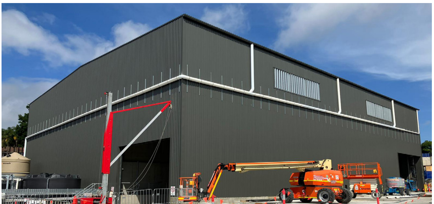
Acoustic shed at the Cammeray site.
