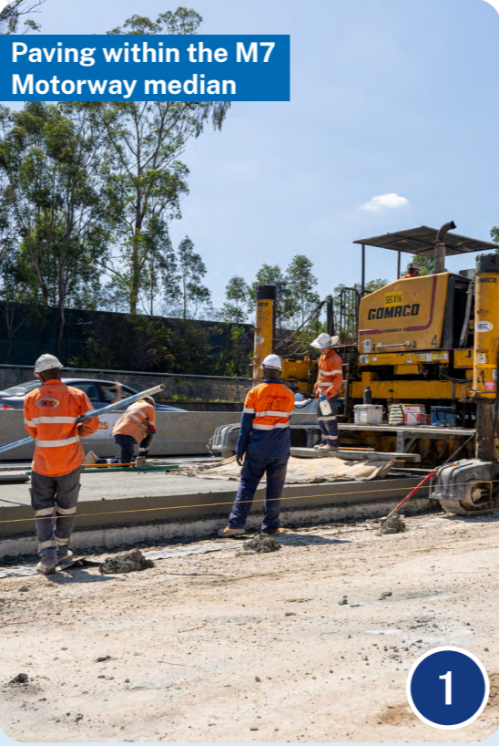
Construction of the new verge within the median
