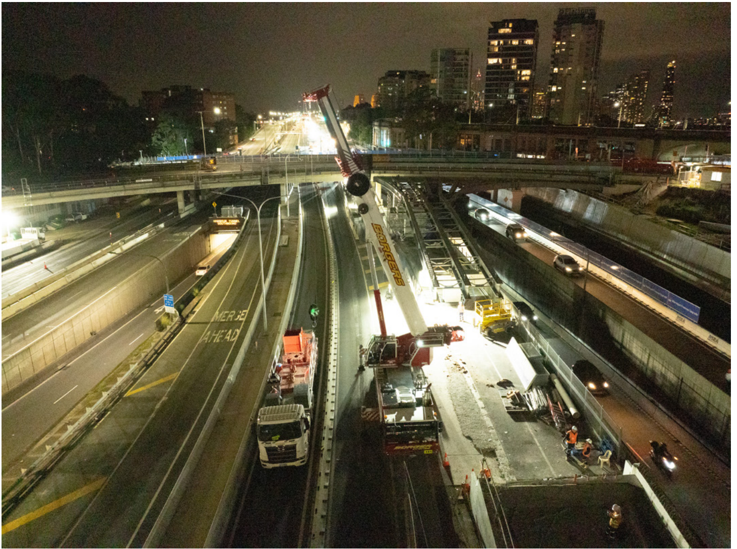
High Street northbound on ramp girders being lifted into place over a weekend of night work in May 2025.
