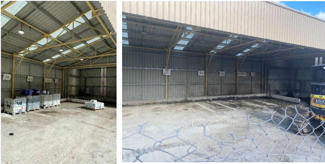
Plate 15-1: Hydrocarbon Waste Storage Yard following upgrades
