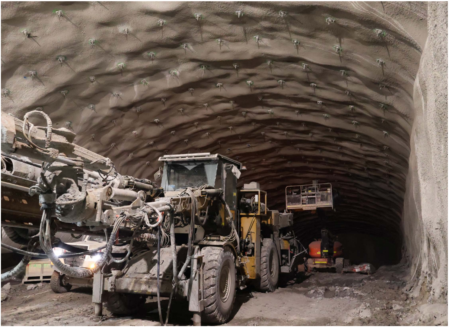
A rockbolter in the Waverton substation for Western Harbour Tunnel.
