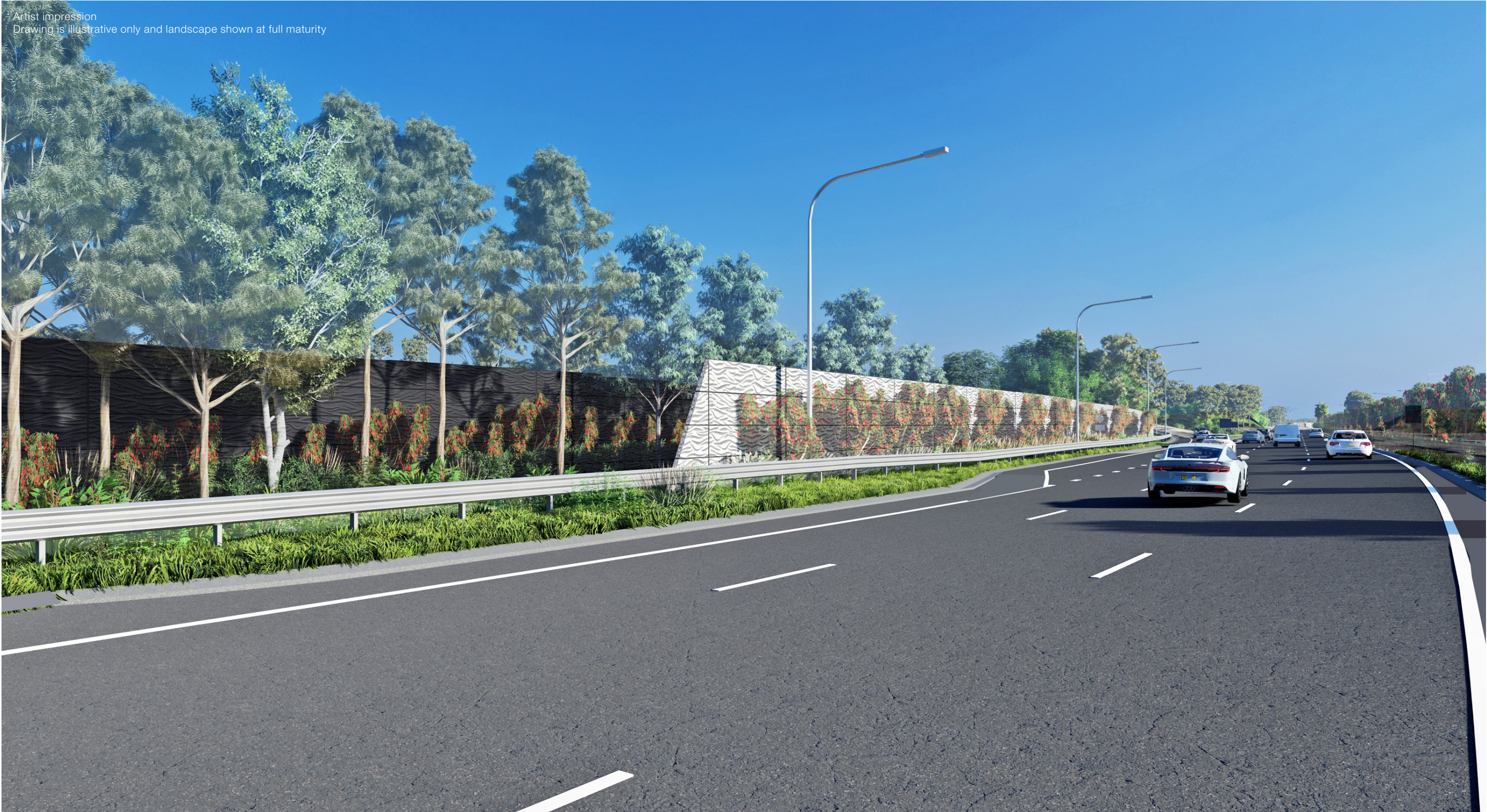
Figure 137: Type 2 RMP noise wall at Tarro, looking north
