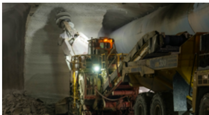
Western Harbour Tunnel Stage 1 roadheader excavation
