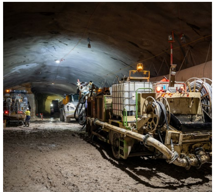
Tunnelling activities at Cammeray
