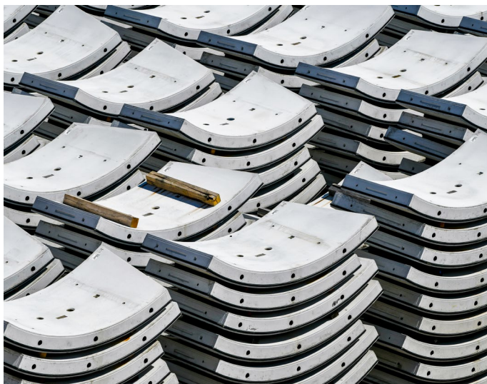
Pre-cast concrete units will fit together to form the tunnel.
