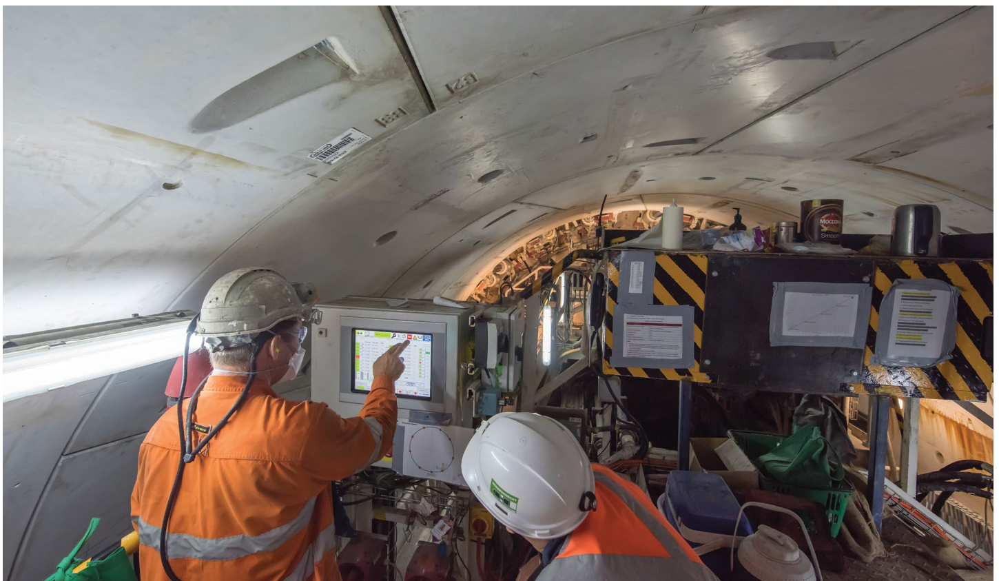
Inside a Tunnel Boring Machine.
