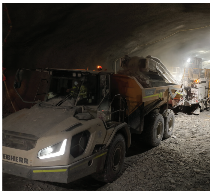
Loading excavated tunnel material for removal (Ridge Street site)
