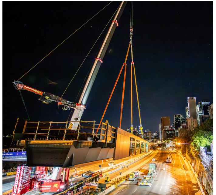
June 2024 - Weekend work at Ridge Street shared user bridge, North Sydney
