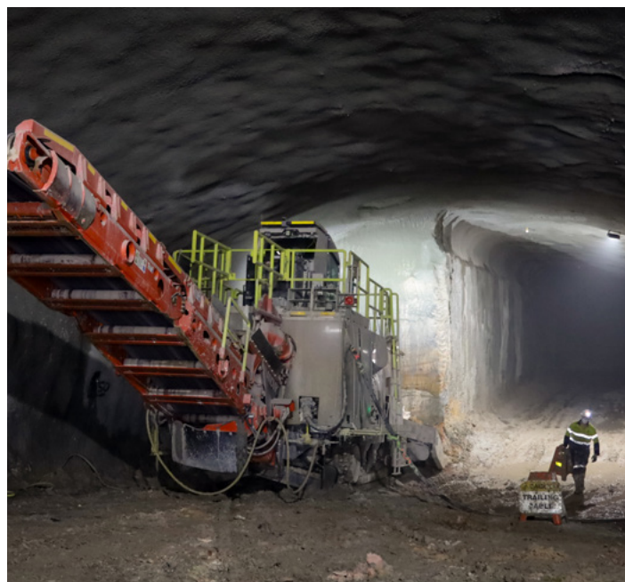
Roadheader tunnelling under Birchgrove launch caverns
