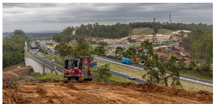
Construction activities taking place for M12 Interchange (facing south)
