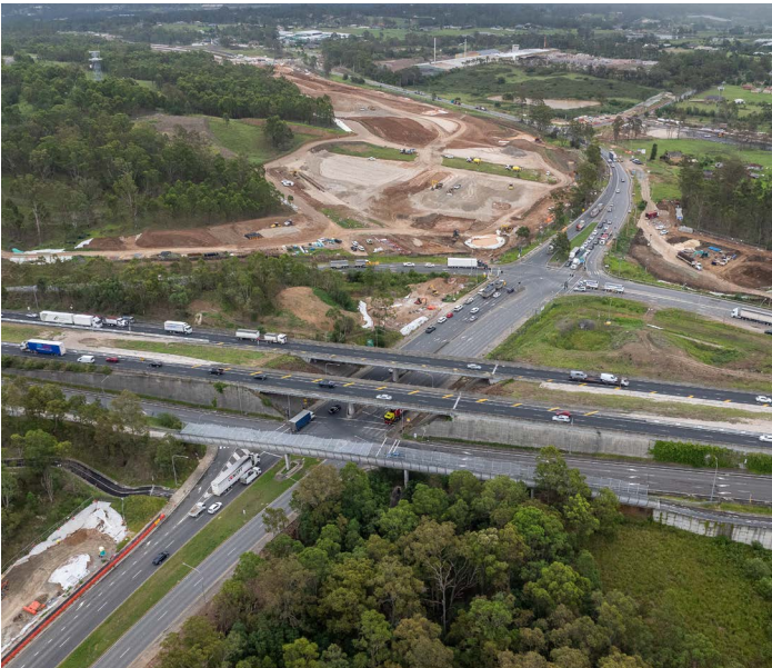
EDC/M12 Interchange (facing west)
