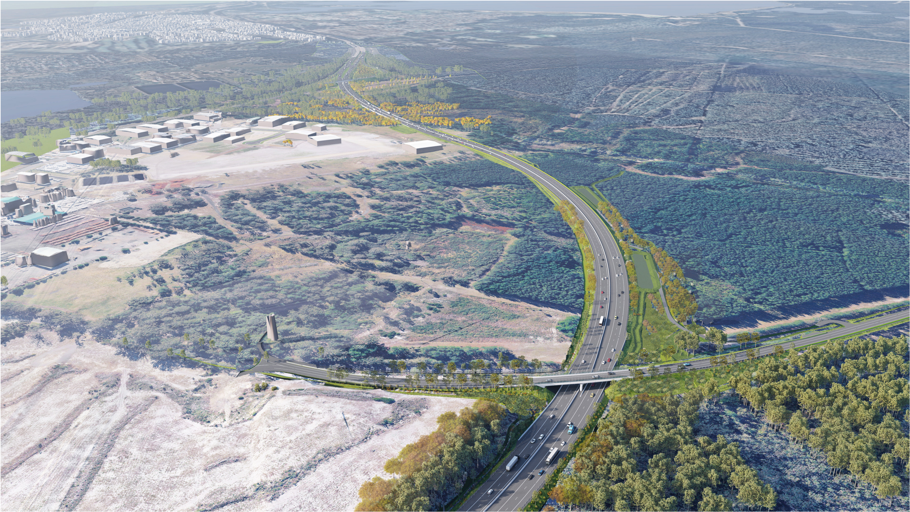
Figure 58: Aerial view of BR10 and Masonite Road
