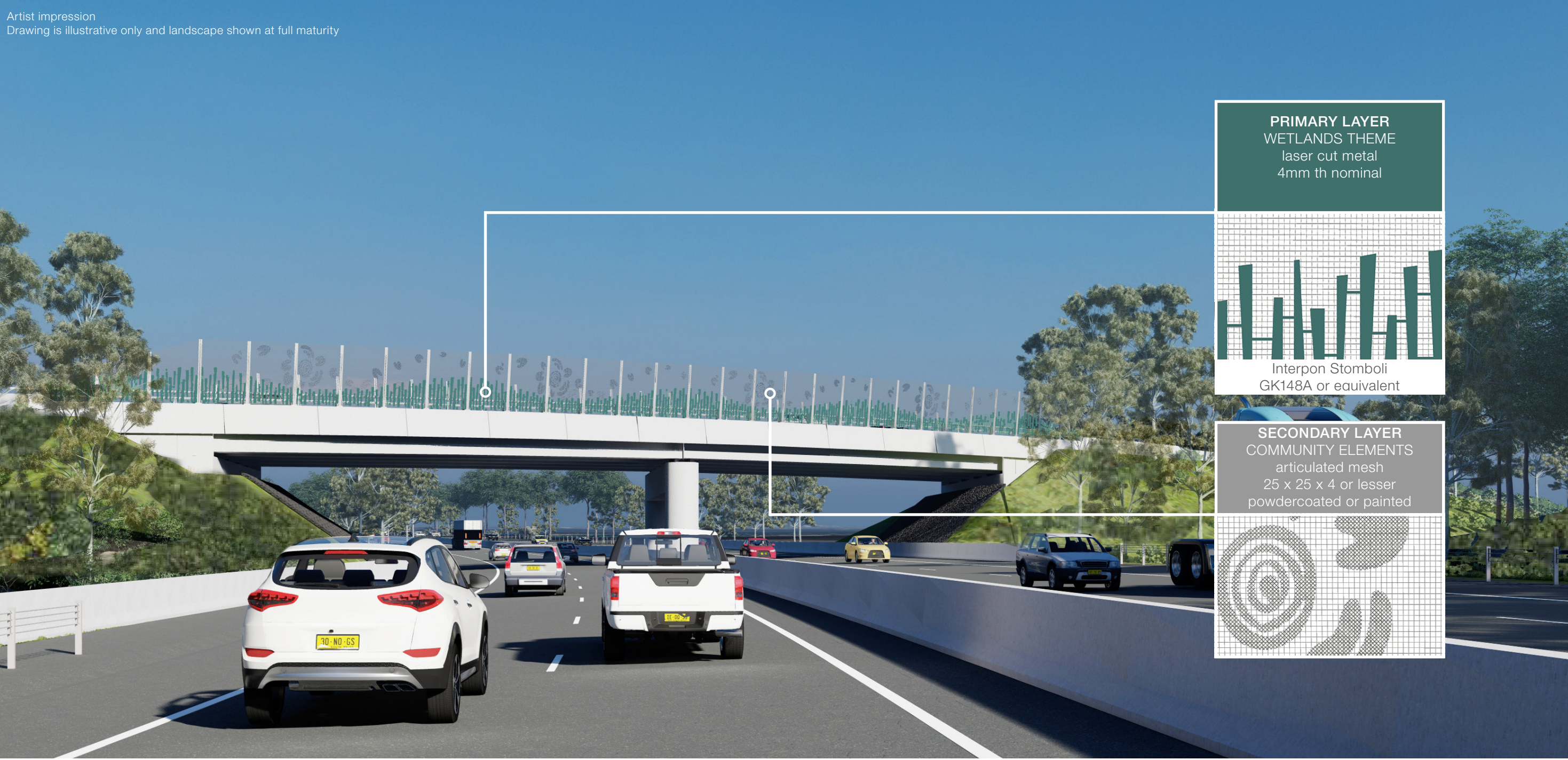
Figure 52: Safety screens - materials
