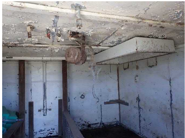
Figure 6-32 Building 11, interior, including ceiling.
