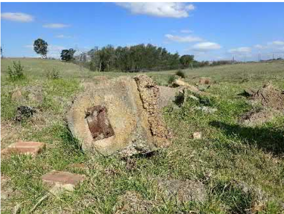
Figure 6-35 Concrete feature, facing east.
