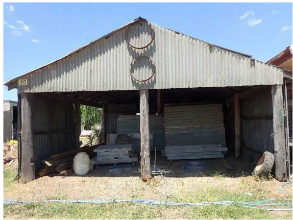
Figure 6-30 Building 9, facing south.
