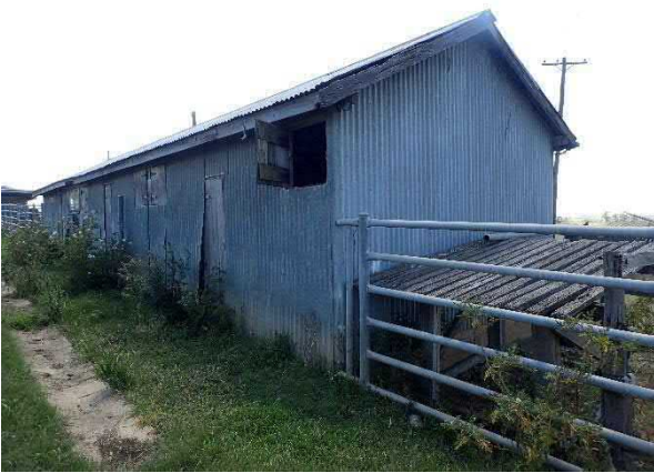
Figure 6-29 Building 5, facing north.
