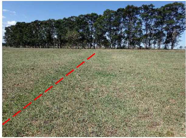
Figure 6-34 Constructed ditch with grove of trees in background, facing east.
