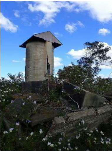
Figure 6-3 Silo and concrete remnants, facing west.
