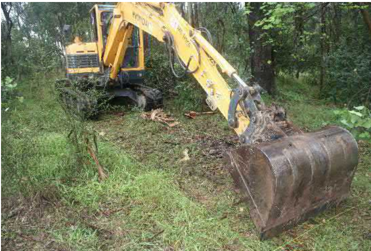
Figure 5-19 Test Trench 5, start of excavation, facing north.
