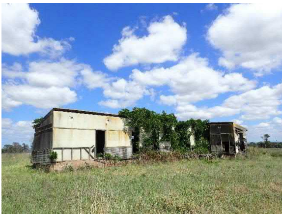
Figure 6-1 Farm 1, facing northwest.
