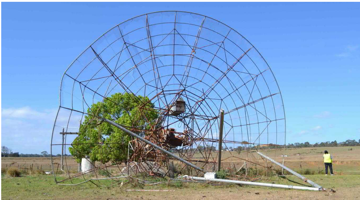
Figure 24 South Creek 2 Antenna Complex: antenna looking east.
