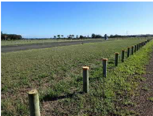
Figure 6-58 Existing bitumen runway (disused) facing north.
