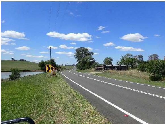
Figure 6-14 Luddenham Road, western road reserve, facing north.
