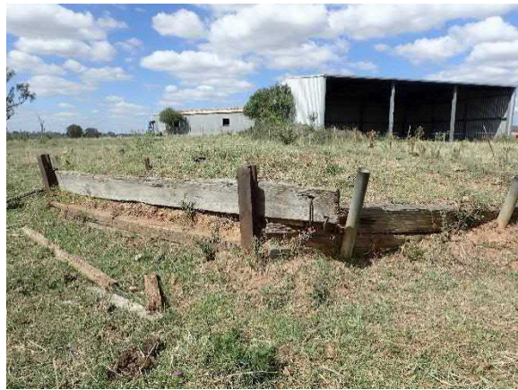
Figure 6-6 Shed 2, in background, facing south.
