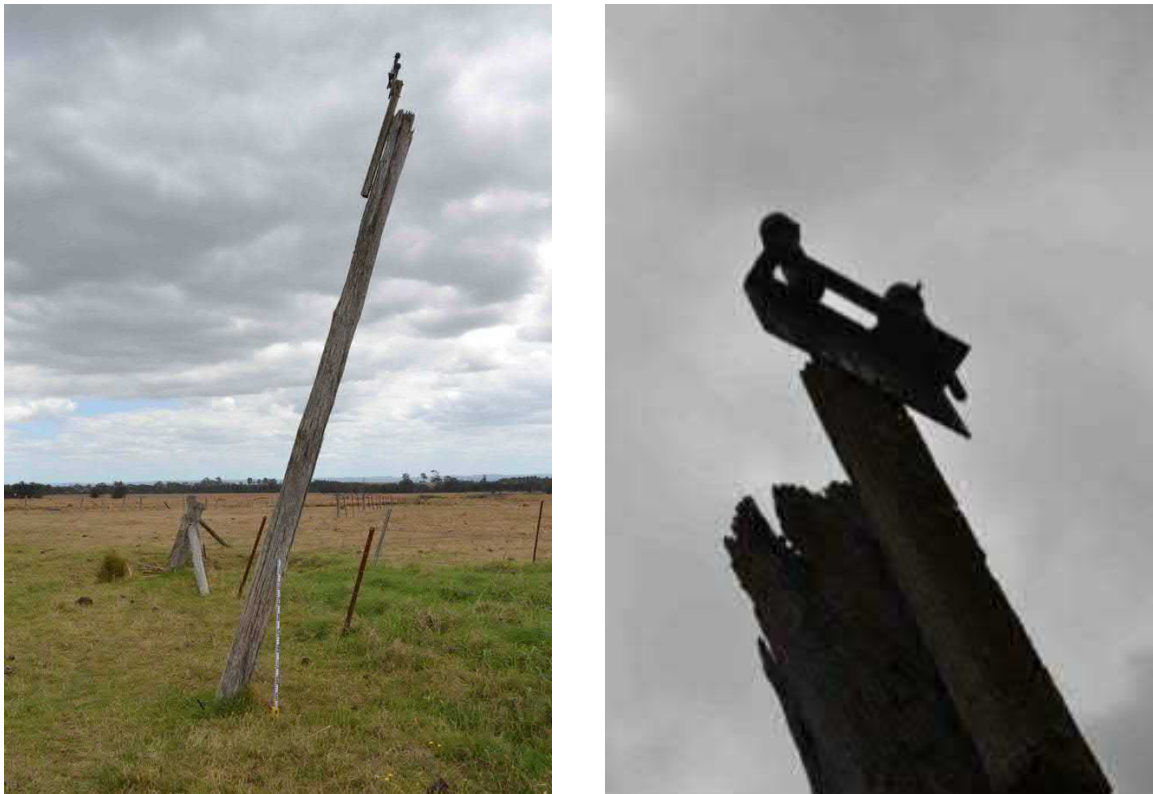
Figure 37 Shain Cross SC02: (left) general view; (right) detailed view.
