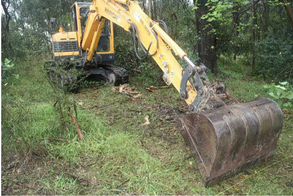
Figure 6: Test Trench 5 – start of excavation
