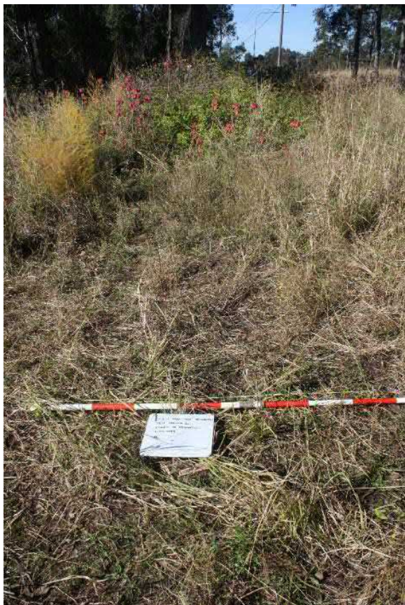
Figure 5-1 Test Trench 1, pre-excitation, facing south-east.
