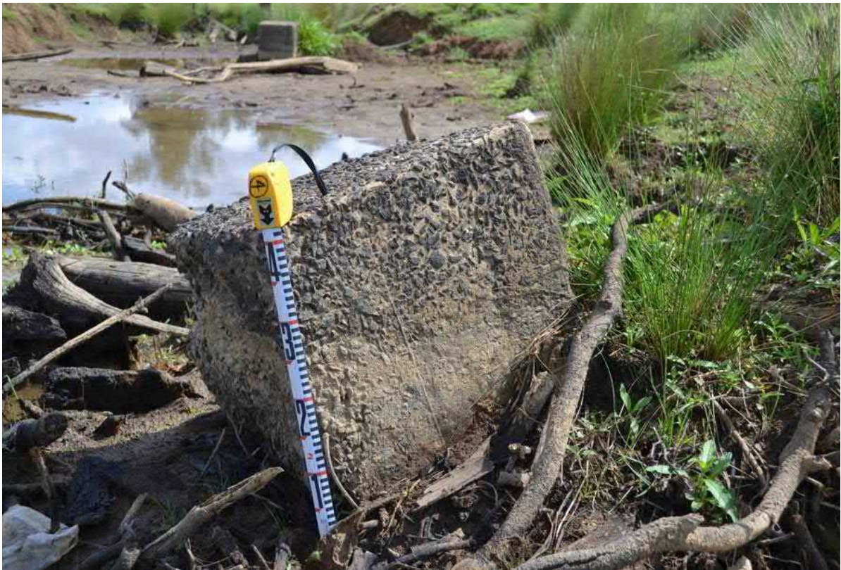
Figure 22 South Creek 1 Antenna Complex: plinths.
