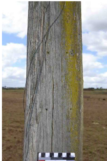
Figure 35 Shain Cross SC01 showing possible switch box attachments.
