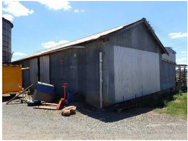
Figure 6-28 Building 4, facing northeast.
