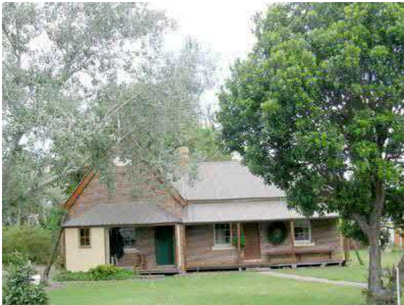
Figure 3-5 Street frontage of the former Agnes Banks Public School (Davies 2005 ).
