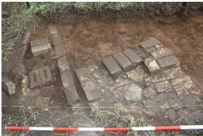
Figure 6-66 Test Trench 1, south-east corner showing the brick and concrete pad [C022] and associated footings [C016, C023].
