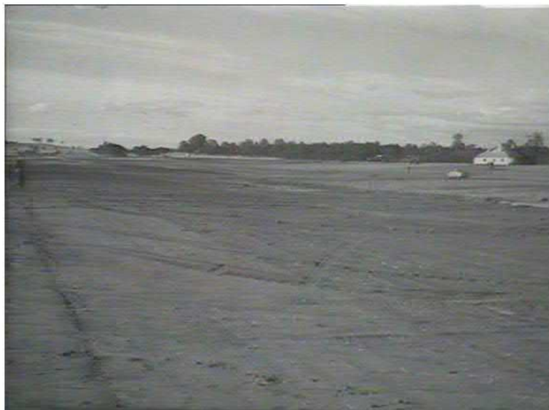
Figure 6-38 Fleurs Aerodrome. Source: Aurecon (2016:137). Originally from State Library of NSW, Government Printing Office 1 – 23753. Main Roads. 'Fleurs Aerodrome – Pan of 2 St25318 to St25319, from south west end 40 degrees runway 50 foot from end 5000 foot peg' date unknown.
