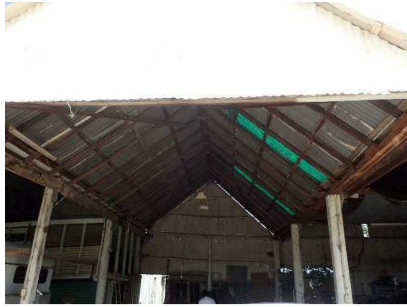
Figure 6-74 Interior of shed, facing east.
