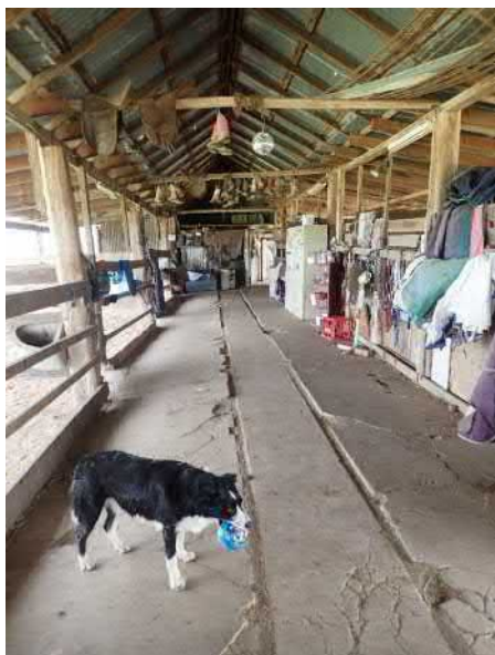
Figure 6-71 Interior of shed, showing rail and timber beams.
