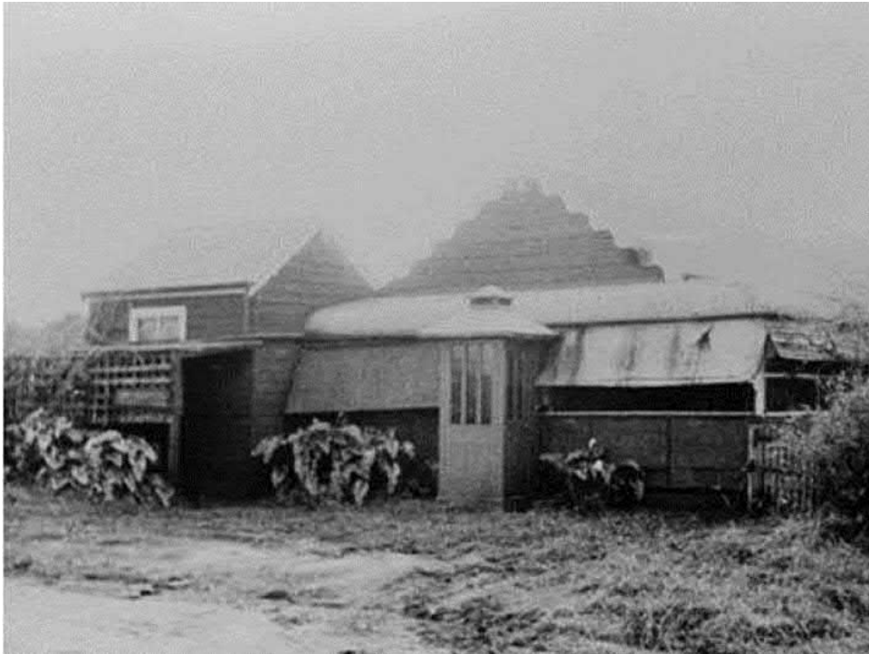
Figure 6-62 Cecil Park Post Office, 1950
