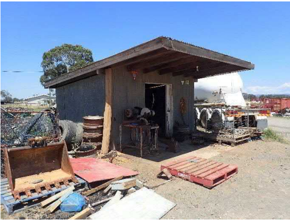
Figure 6-27 Building 3, facing south.
