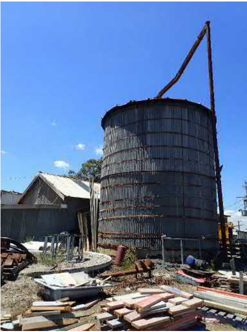
Figure 6-33 Silo 1, facing southeast.
