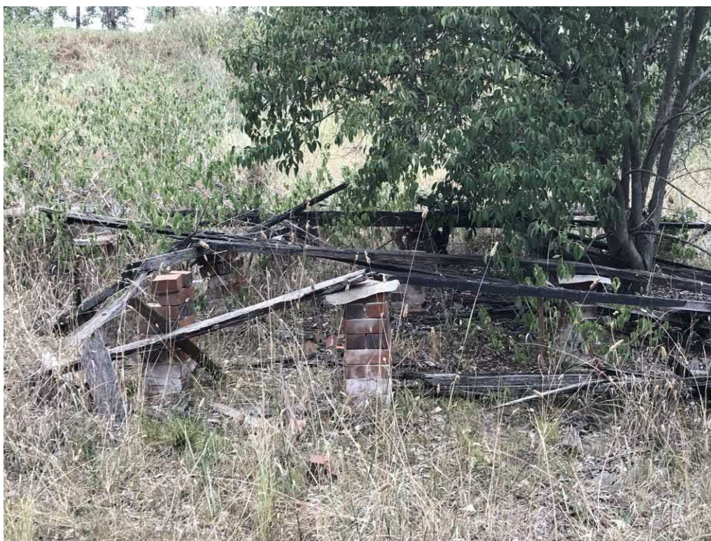
Figure 6-91 Northern end of former Public Hall, looking east towards Wallgrove Road. A small set of concrete stairs is located to the right (out of frame)
