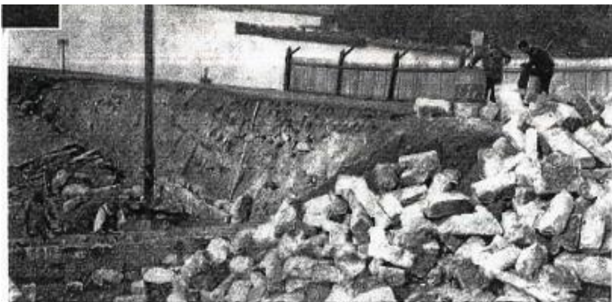
Figure 3-4: Sandstone blocks from the warehouse being laid for the bund wall in the 1930s (taken from AMAC 1999)
