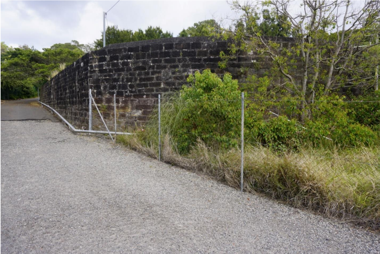
Figure 3-8: The bund wall in the southwest corner of the project site. View to the northwest.
