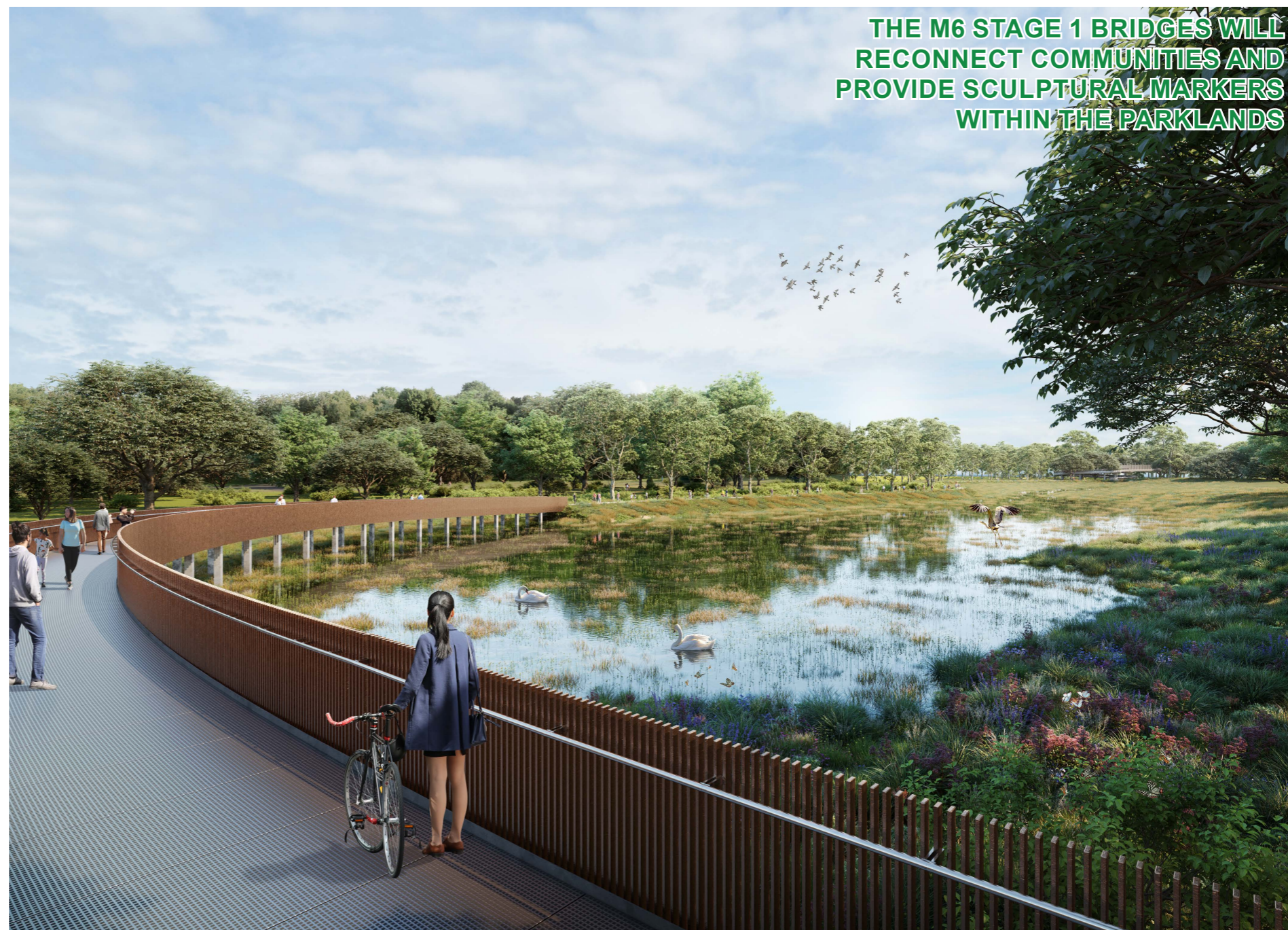
Artist's impression - Bridge over Scarborough Ponds (existing condition shown indicatively). Trees and landscape shown at maturity.
